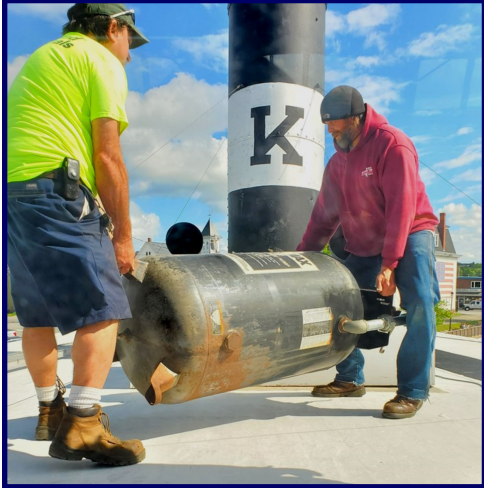
Everyone knows the sound of Kate's whistle! Captains Randy Gartley and Matt Kane install a new whistle tank for the Katahdin in preparation for the 2022 cruising season. Thank you to the Town of Greenville for the whistle tank.
