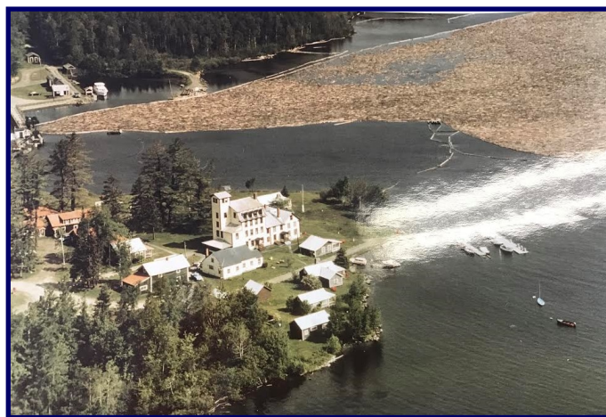
Log boom at East Outlet and Wilson's Camps.
