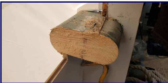
Katahdin's "Green Rail" before demolition.
